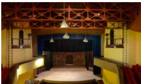
Steel roof construction in theatre hall
