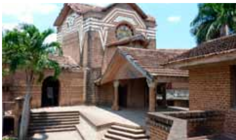
View of the theatre building from outdoor balconies (9) of the dancehall
