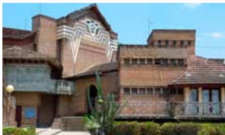
Entrance to reception and offices on Avenida 26 de Julio
